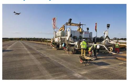
After years of pursuing planning permission to build an all-weather runway at Sywell Aerodrome, consent was awarded in April 2008 to build the 1.5km, 30m wide runway at this historic site. Laing O'Rourke were engaged in May 2008 to deliver the concrete paving for the new runway
